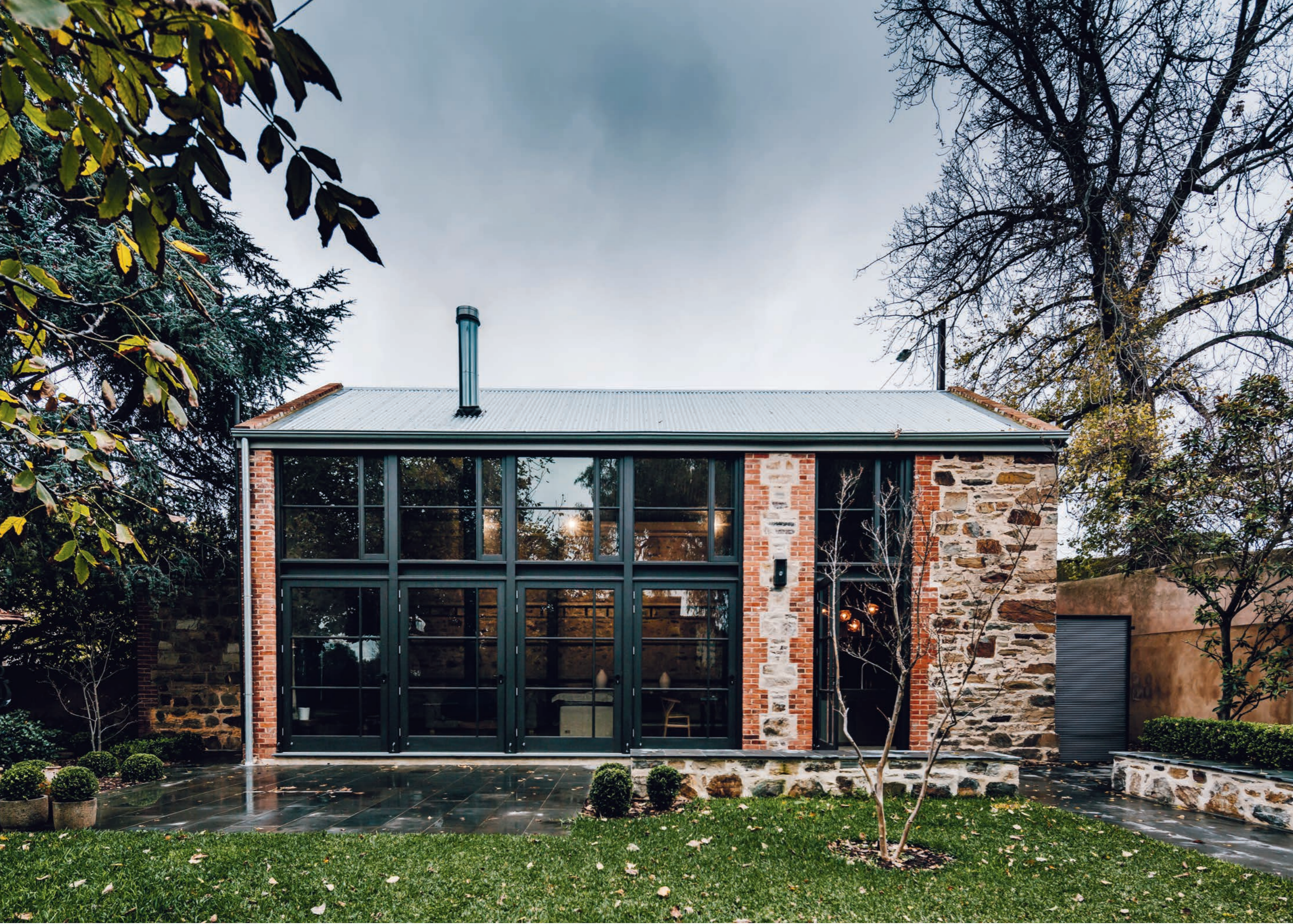
NORTH ADELAIDE BARN ADELAIDE, SOUTH AUSTRALIA
